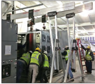
Contractor used 2-11000R Gantry Cranes to move 16000 lb. electrical cabinets on Third floor of assembly hanger. Job was on time, under budget
