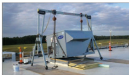
4400T Gantry Crane lifting 3500 lb. A/C unit on roof of building. Job took 2 hours, saved contractor $20,000 in crane costs
