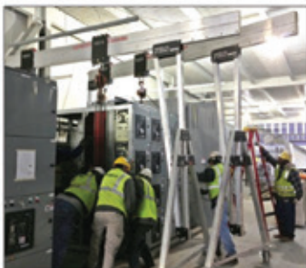
Contractor used 2-11000R Gantry Cranes to move 16000 lb. electrical cabinets on Third floor of assembly hangar. Job was on time, under budget
