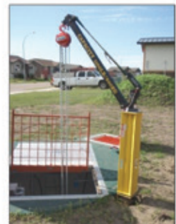
1100 lb. capacity Davit Crane servicing neighbourhood pump station
