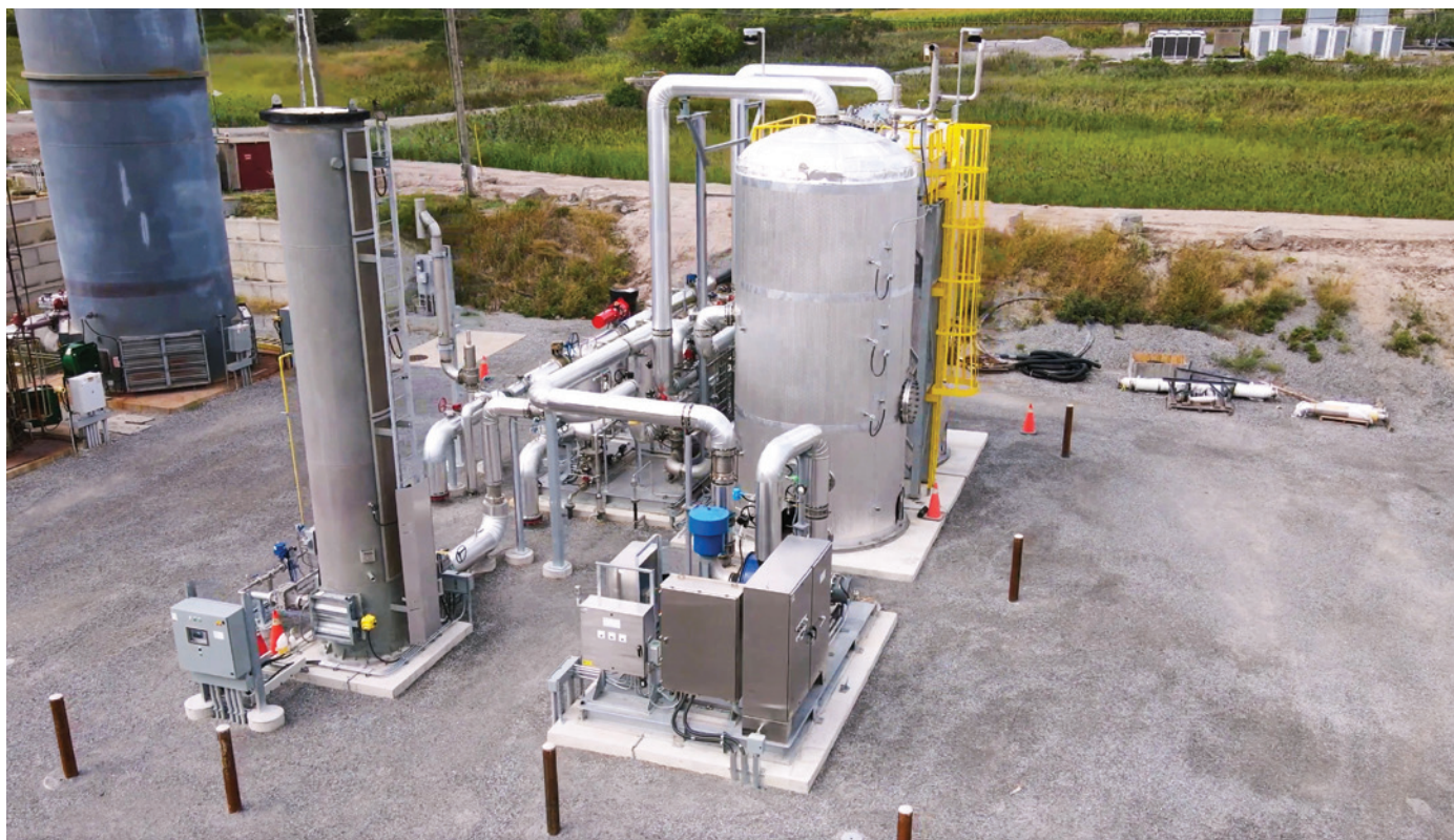
Renewable landfill gas will power 35% of GM's electrical demand at its St. Catharines Propulsion Plant, while cogenerating significant heat for the facility.
